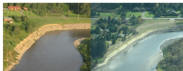
► Before and after pictures of a bank stabilization project - Little Main Restigouche River
